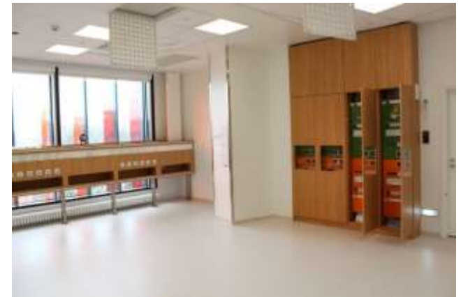
Photos: MEV-system in The New Children's Hospital in Helsinki.
